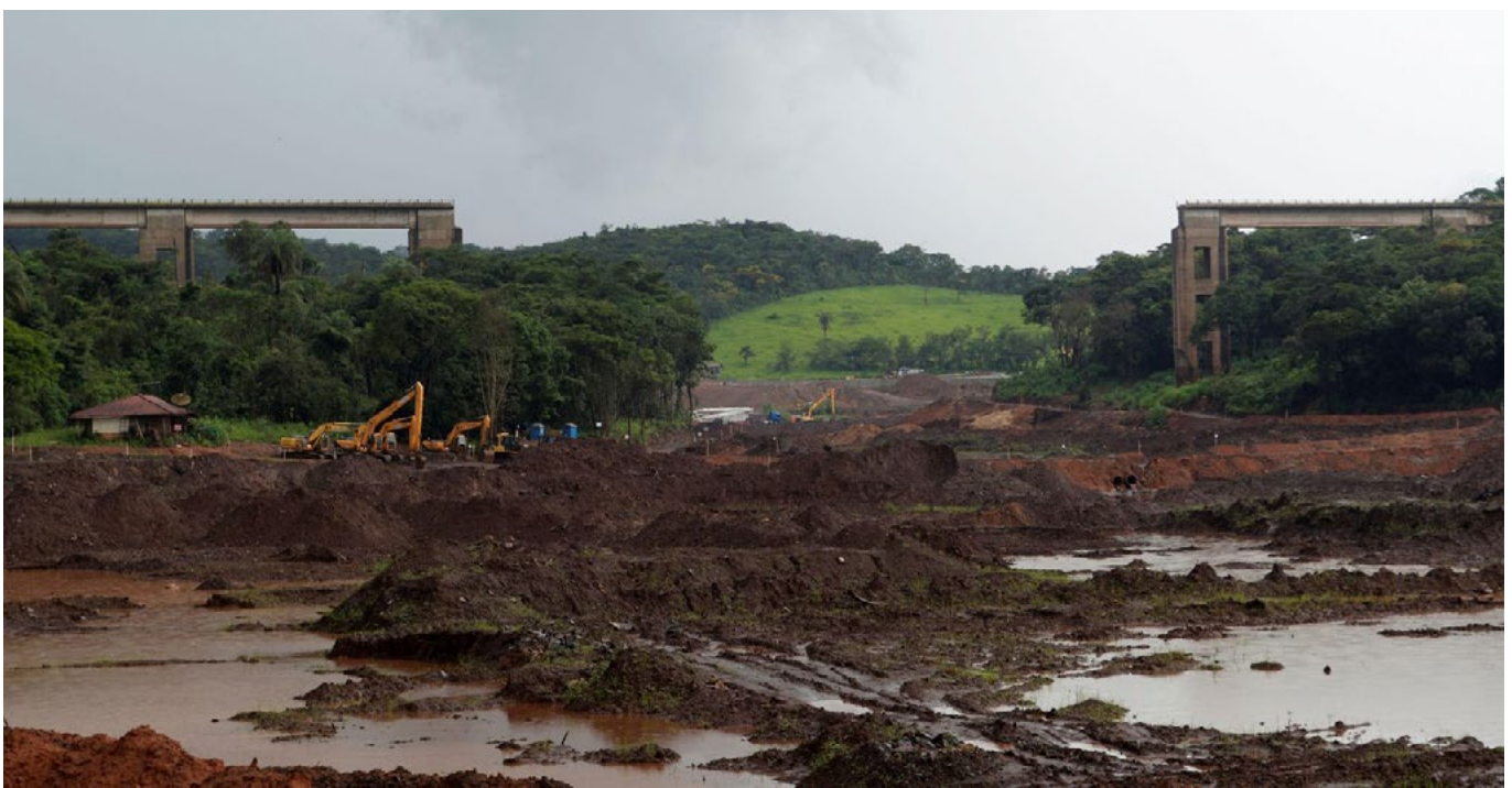
Vale's tailings dam in Brumadinho
